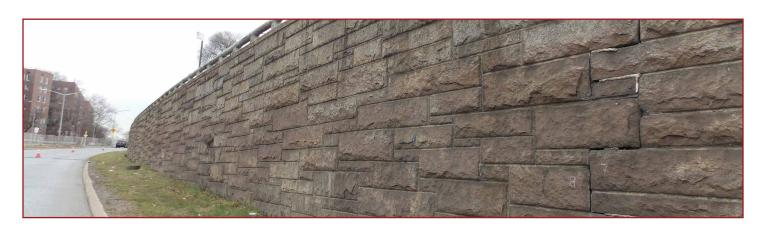
NYSDOT Contract D038186: Retaining Wall Inspections and Corrective Maintenance, New York, NY | The project scope included the enhanced hands-on and visual inspection of priority walls on all NYSDOT-owned retaining walls along arterial highways / locations and in-depth inspection of walls with defects. KC's geotechnical group
