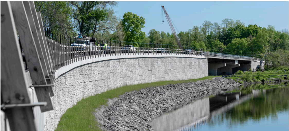
On NYSDOT's D900034 Region 8 Bridge Replacement DB, KC, as Lead Designer, provided the design of the two bridge structures, including staged construction and WZTC; geotechnical work; environmental permitting; surveying; roadway design; hydraulic analysis; and quality management services.
