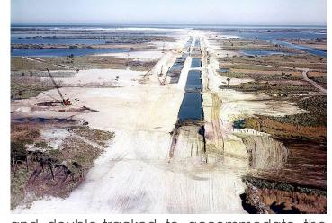
and double-tracked to accommodate the Crawler-Transporter. Resembling a highway, the 2 lanes are 40 feet wide and separated by a median that is 50 feet wide. But while highways are designed to carry the weight of cars, trucks, and other ordinary vehicles, the Crawlerway was designed to carry a live load of up to 26 million pounds: enough to accommodate the combined weight of the Saturn V rocket and its Crawler-Transporter, which equated to roughly 17 million pounds.
