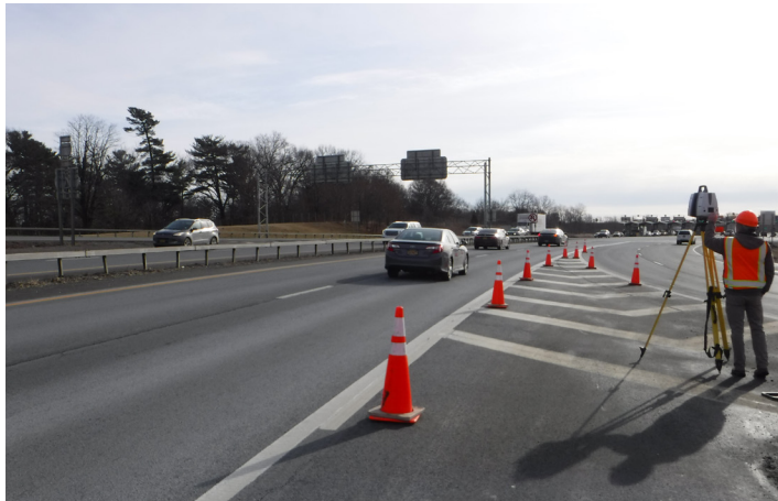
KC personnel surveying I-87, part of the Interstate Highway System.
