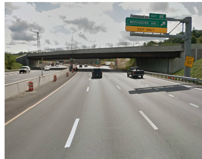
The Cross-Westchester Expressway (I-287)
