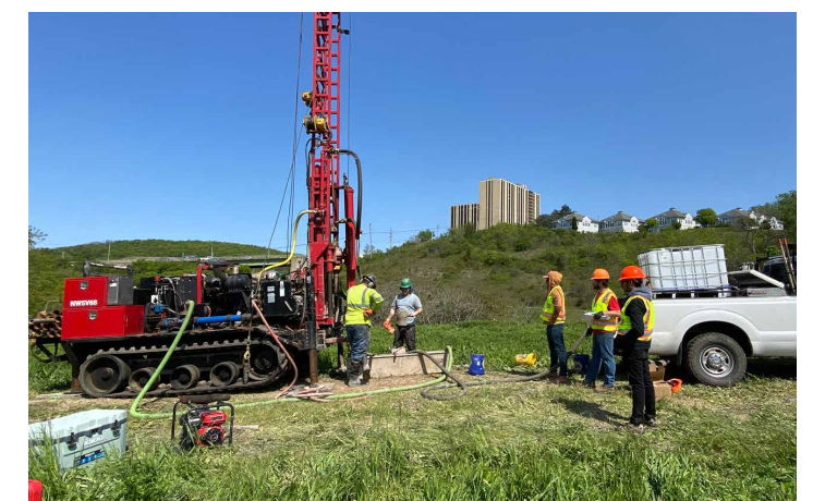
KC recently started work as Lead Designer and Quality Manager for the NYSDOT I-81 Viaduct Phase 2, Contract 6 Design-Build, the largest in NYSDOT history.
