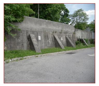
**Municipal Parking Lot, Wappingers Falls, NY** | The Mill Street parking lot has 2 retaining walls, totaling approximately 186 linear feet, of various heights and construction running along the south and east boundary of the property. The east retaining wall height varies from 10' to 14' in height with a 2' to 4' curb reveal. The south retaining wall is approximately 5' in height and ends at grade.
