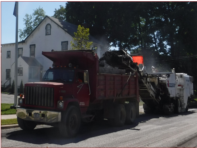
South Avenue Paving
