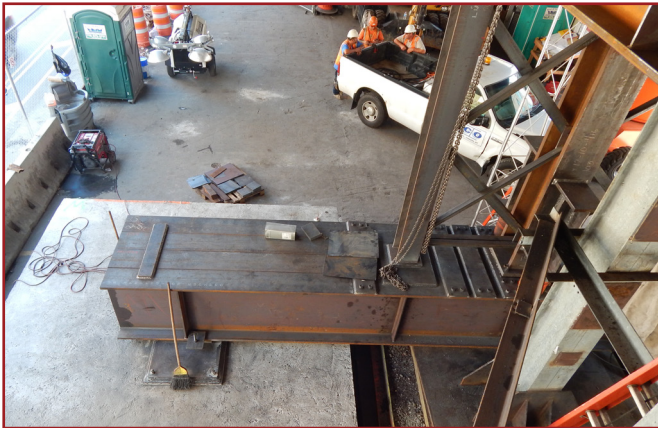
Temporary Support Framing
