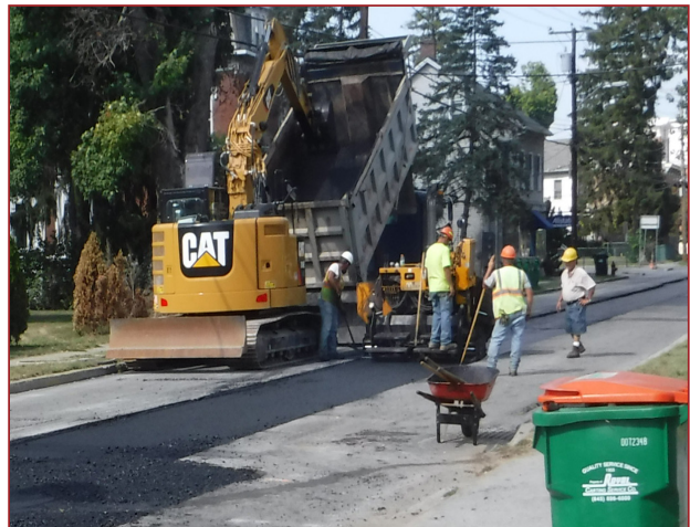
South Avenue Paving
